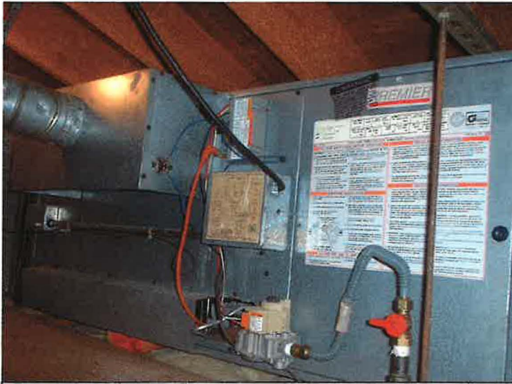
The Gant furnace showed no signs of heat exchanger fatigue, but the model number matched the recall.
