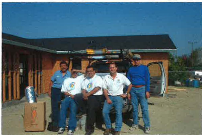
The Mt. SAC crew at 21170 Clover Avenue
