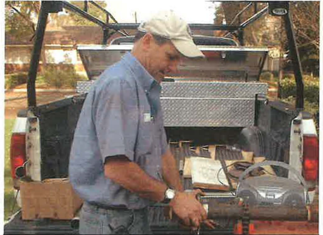
Installing the replacement furnace at the Corydon home
