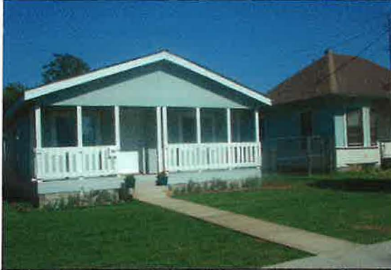
The completed home on Columbia
