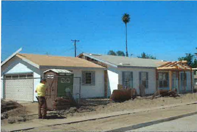
The Dracica house is installed on footings
