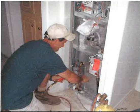
The refrigerant lines are brazed
