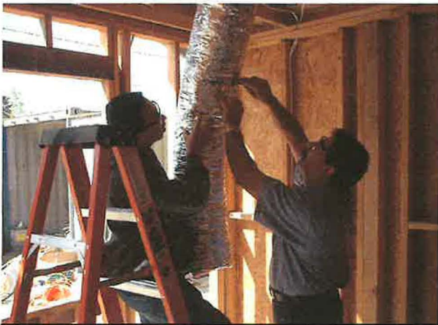
Students installing flex duct for the supply air
