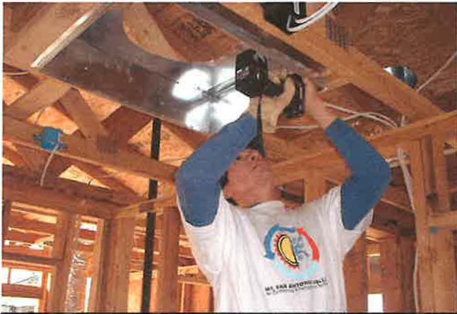
A student installs the return air can
