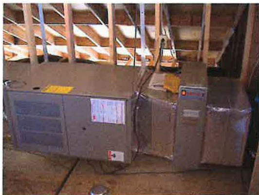
Horizontal furnace installed in the attic
