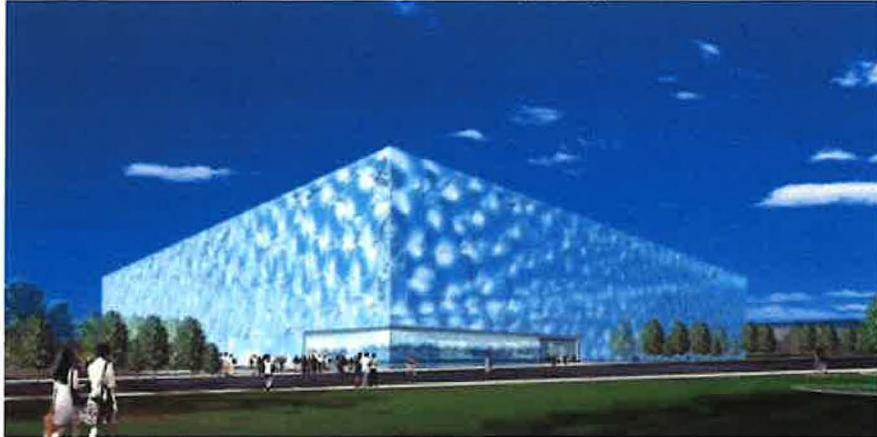
The striking exterior of the National Swimming Center, being constructed for the 2008 Olympic Games and nicknamed, the "Water Cube," is made from panels of a lightweight form of Teflon that transforms the building into an energy-efficient greenhouse-like environment. Solar energy will also be used to heat the swimming pools, which are designed to reuse double-filtered, backwashed pool water that's usually dumped as waste.
