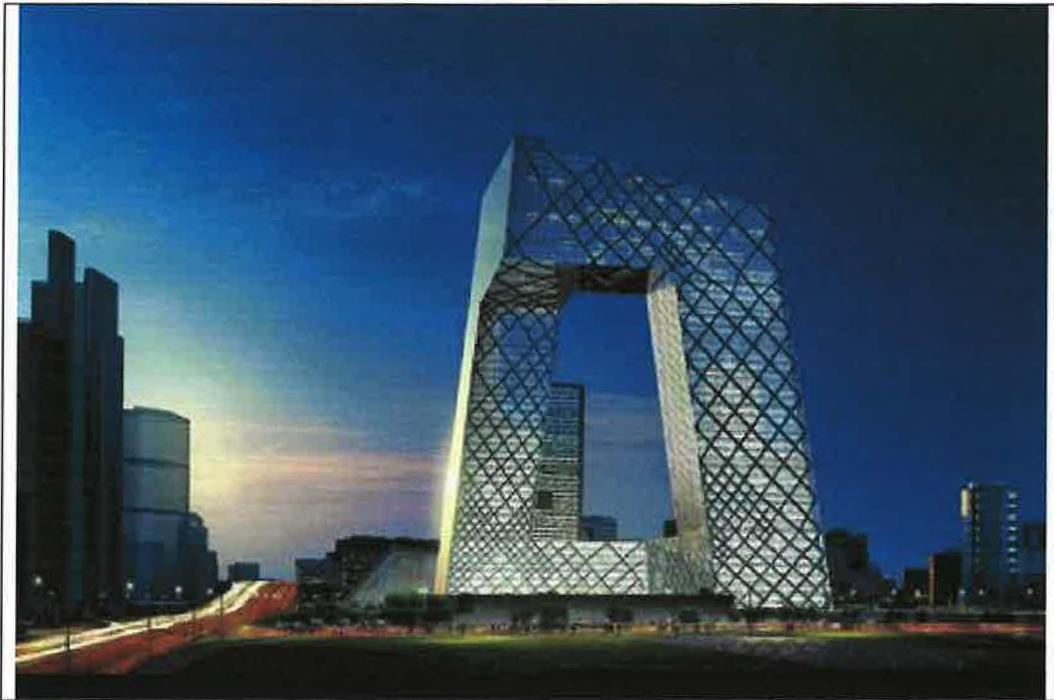
The design of the new Central Chinese Television (CCTV) headquarters defies the popular conception of a skyscraper – and it broke Beijing's building codes and required approval by a special review panel. The standard systems for engineering gravity and lateral loads in buildings didn't apply to the CCTV building, which is formed by two leaning towers, each bent 90 degrees at the top and bottom to form a continuous loop.
